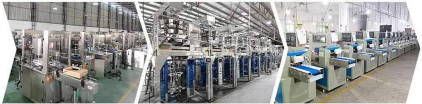
FILLING MACHINE WORKSHOP
