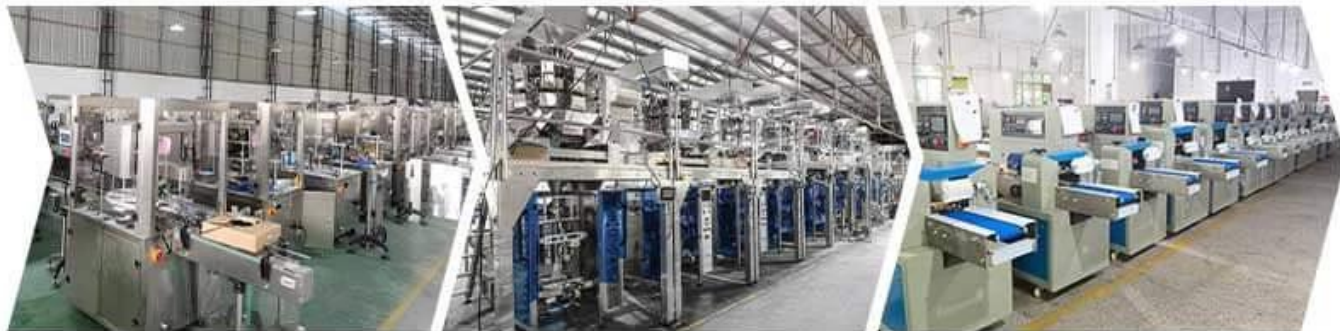
FILLING MACHINE WORKSHOP
